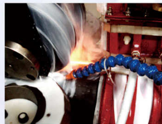
Four Rolls SQ. Welding
